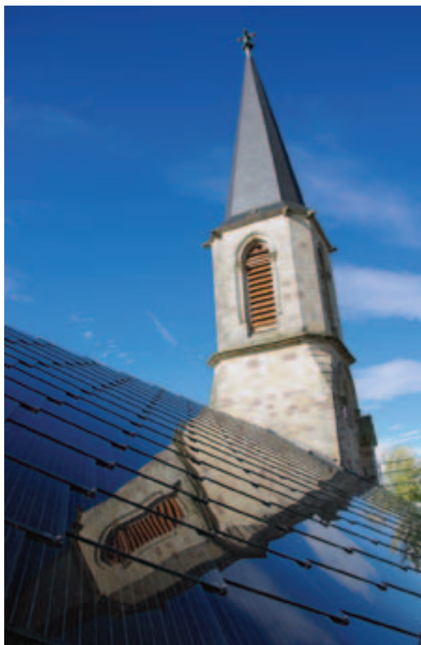
Photo 4.5 Manspach church (Alsace, France) renovated using photovoltaic tiles
