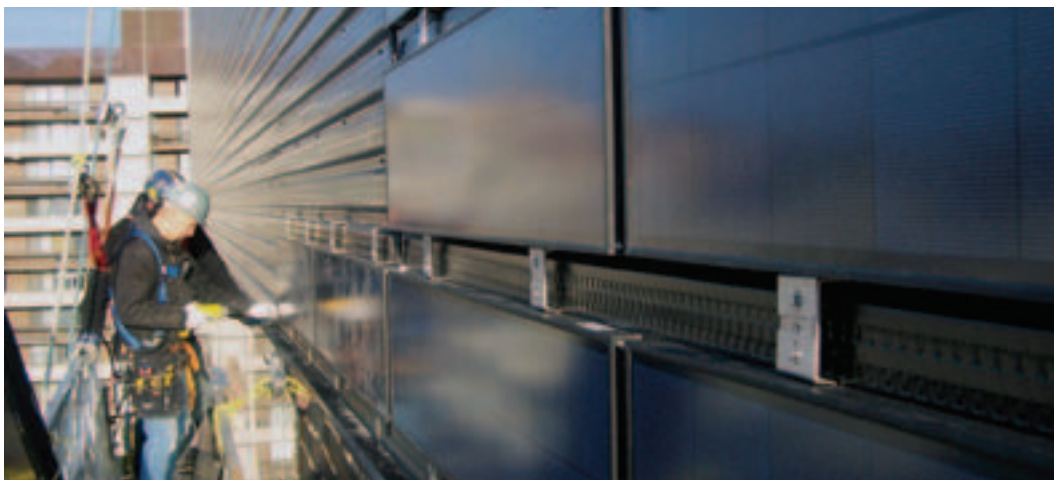
Photo 4.8 Installing a solar air heating system
