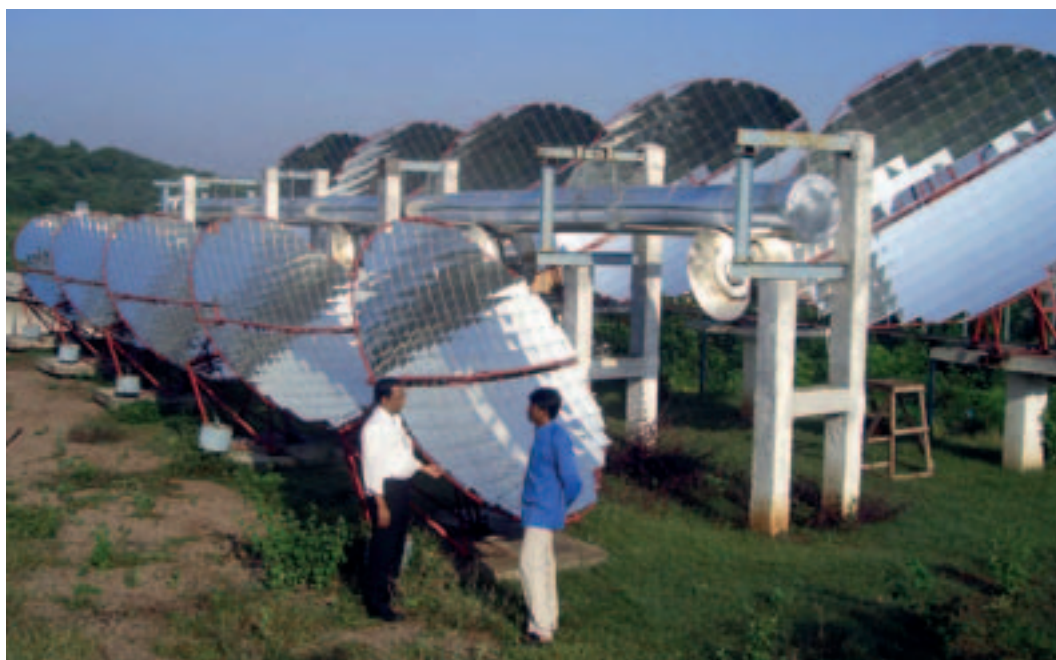
Photo 7.7 Scheffler dishes associated in pairs in a cooking system at Hyderabad (India)
