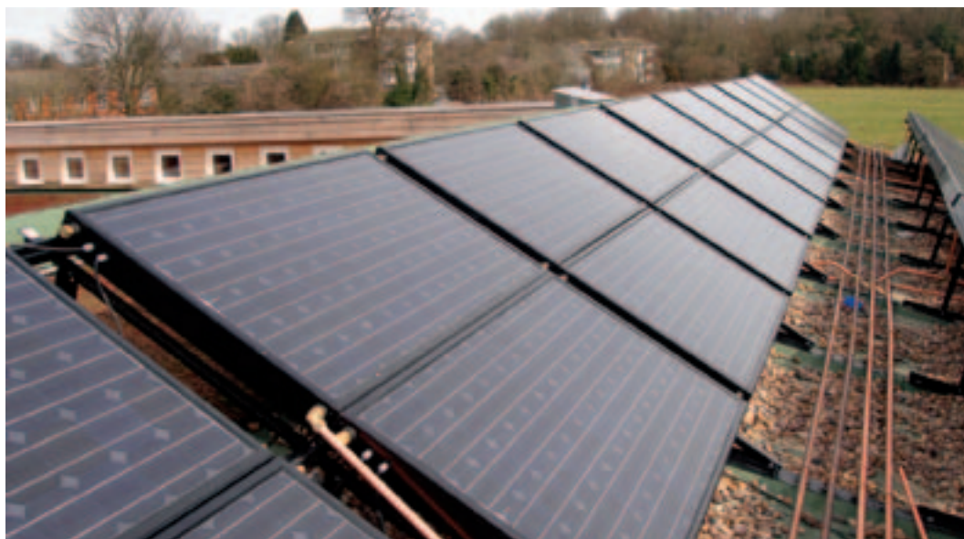
Photo 6.1 PV-thermal collectors manufactured in Turkey
