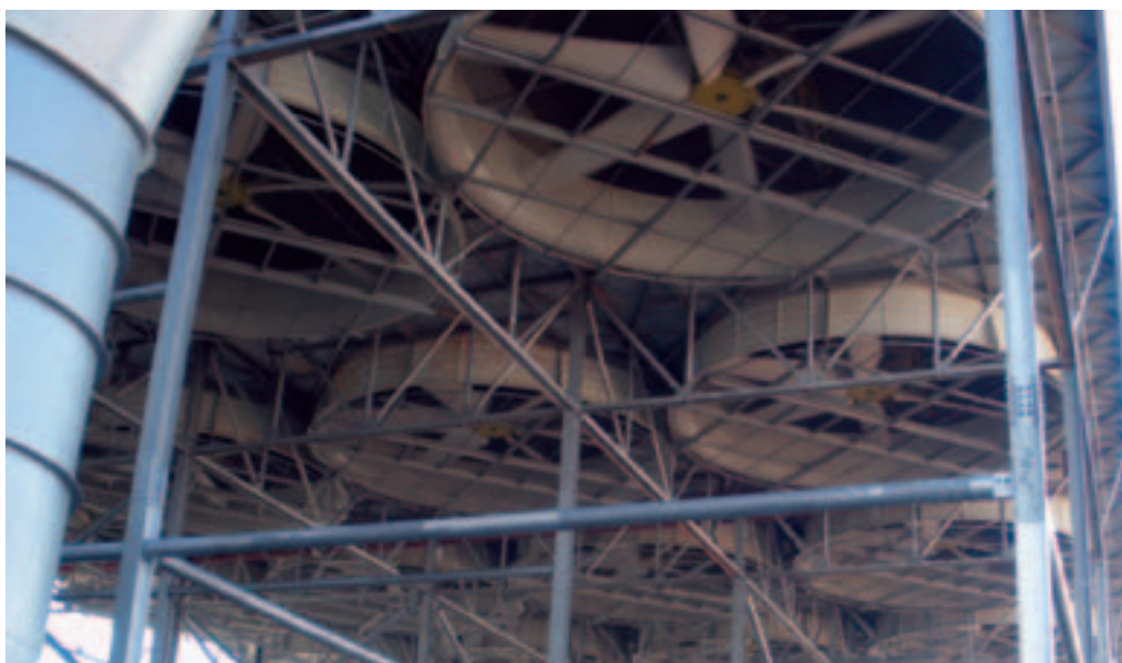
Photo 8.3 Dry cooling of the integrated solar combined cycle plant at Ain Beni Mathar, Morocco
