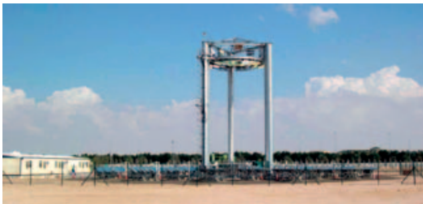
Photo 7.8 Experimental beam-down solar tower in Abu Dhabi
