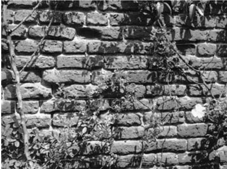
Figure 6.14 A fairly common defect caused by shrubs sending their roots into brick joints
