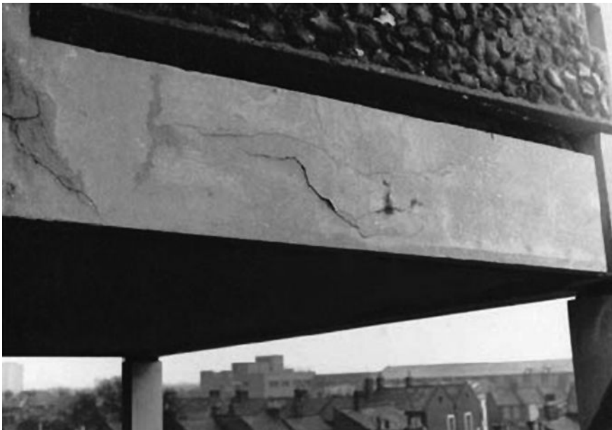
Figure 7.2 Corrosion of reinforcement causing cracking of concrete. Reproduced by permission of Harsco Infrastructure
