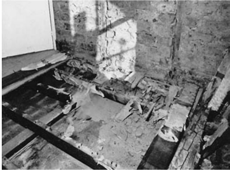
Figure 9.1 Dry rot spore dust in floor joists and partition. Reproduced by permission of Harsco Infrastructure
