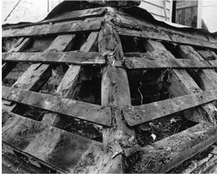
Figure 10.11 Timber roof structure after worn stone slates have been removed
