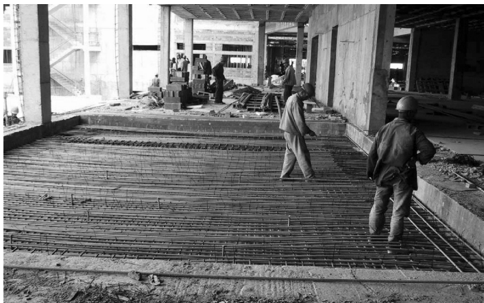
Figure 1.10 GFRP reinforced-concrete slab (Oran, Algeria).
