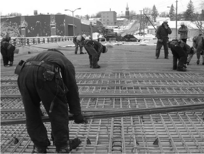
Figure 1.6 GFRP reinforced-concrete bridge deck (Cookshire-Eaton, Quebec, Canada).
