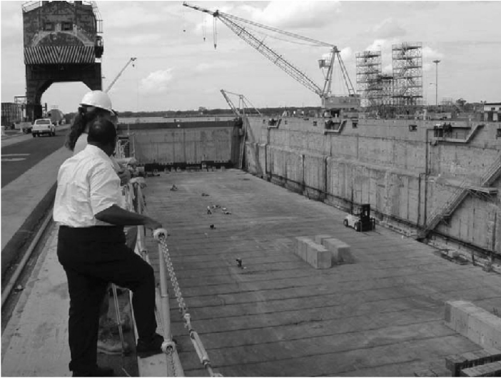
Figure 1.4 GFRP reinforced-concrete repair for Pearl Harbor dry docks (Honolulu, Hawaii).
