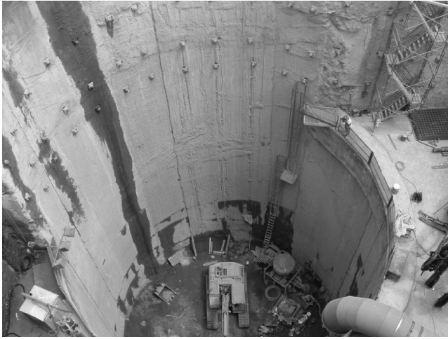
Figure 1.14 GFRP reinforced-concrete soft-eye for Beacon Hill light rail transit (Seattle, Washington).
