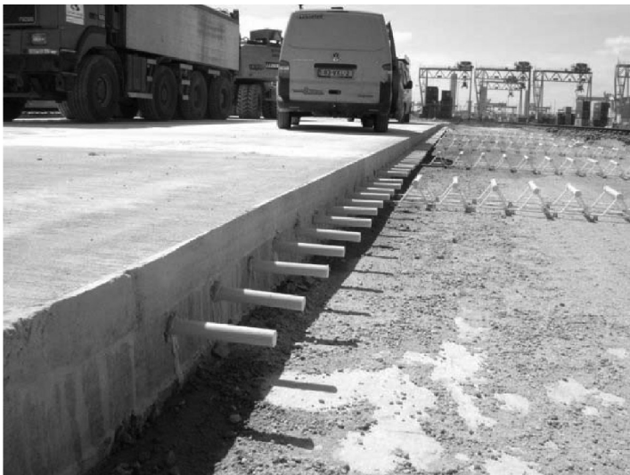
Figure 1.3 Dowel bars in concrete pavements (Port of Rotterdam, The Netherlands).
