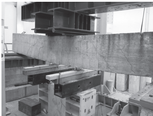
(a) Immediately prior to failure with marked-up cracks
