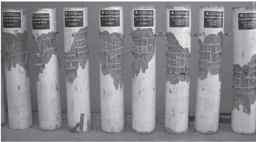
(c) Column specimens after failure
