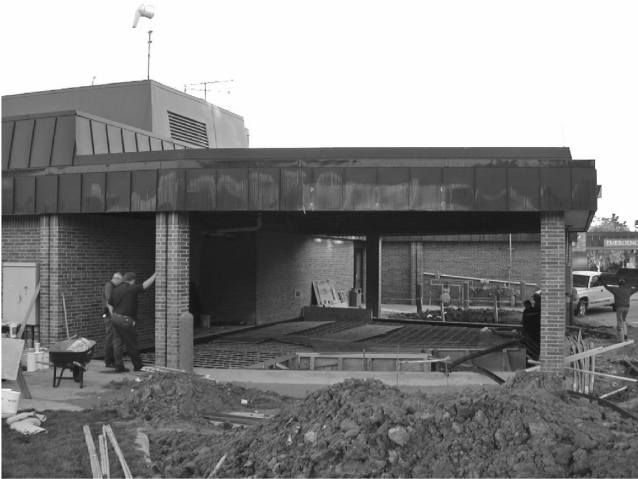
Figure 1.9 GFRP reinforced-concrete slab for MRI rooms in hospital (York, Maine).
