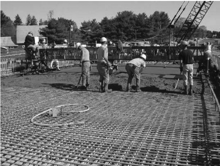
Figure 1.5 GFRP reinforced-concrete bridge deck (Morristown, Vermont).
