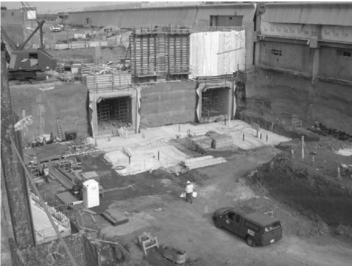
Figure 1.13 GFRP reinforced-concrete soft-eye for Washington Dulles International Airport people mover (Dulles, Virginia).
