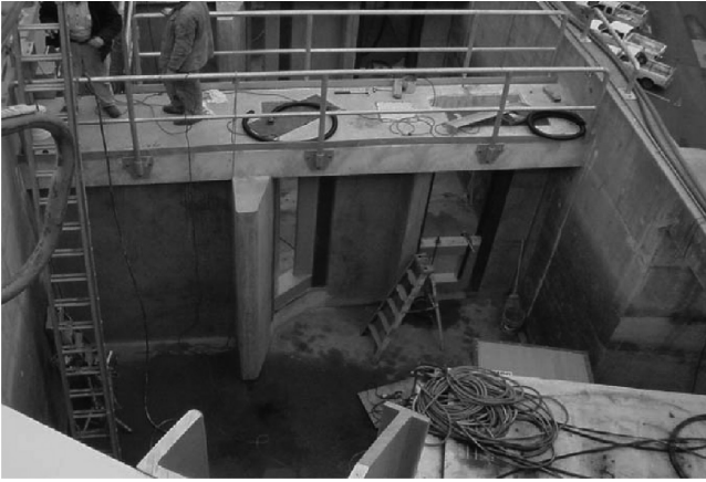
Figure 1.8 GFRP reinforced-concrete for Ice Harbor lock and dam fish weir (Walla Walla, Washington).
