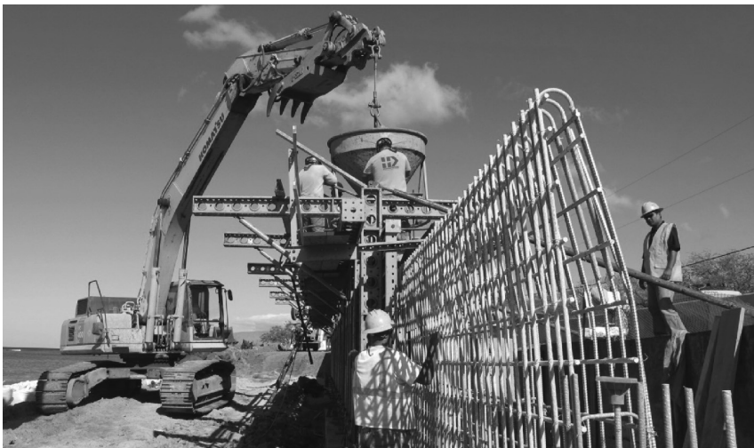
Figure 1.2 Honopapiilani highway retaining sea wall south (Lahaina, Maui Hawaii).
