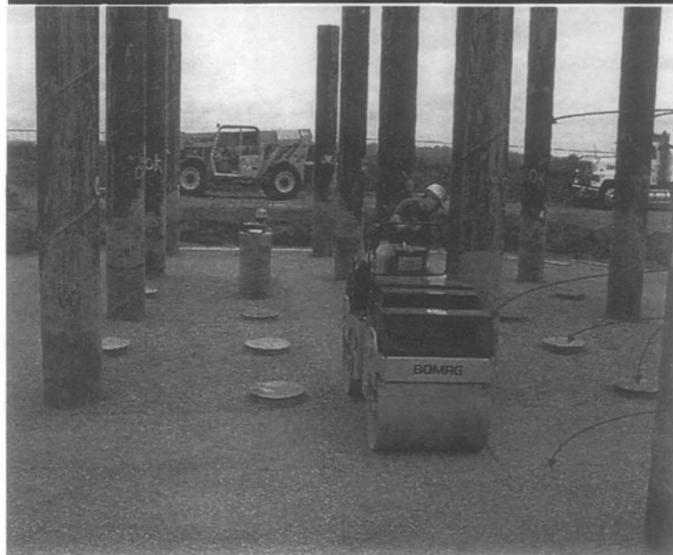
Figure 47-1 Compacting the gravel housekeeping mat.
