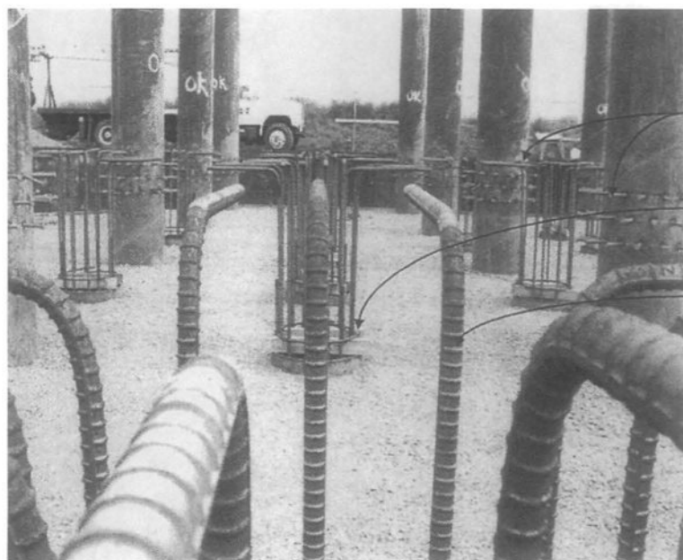
Figure 47-2 This is a view of pile columns above grade and pile columns with rebar cages at grade.
