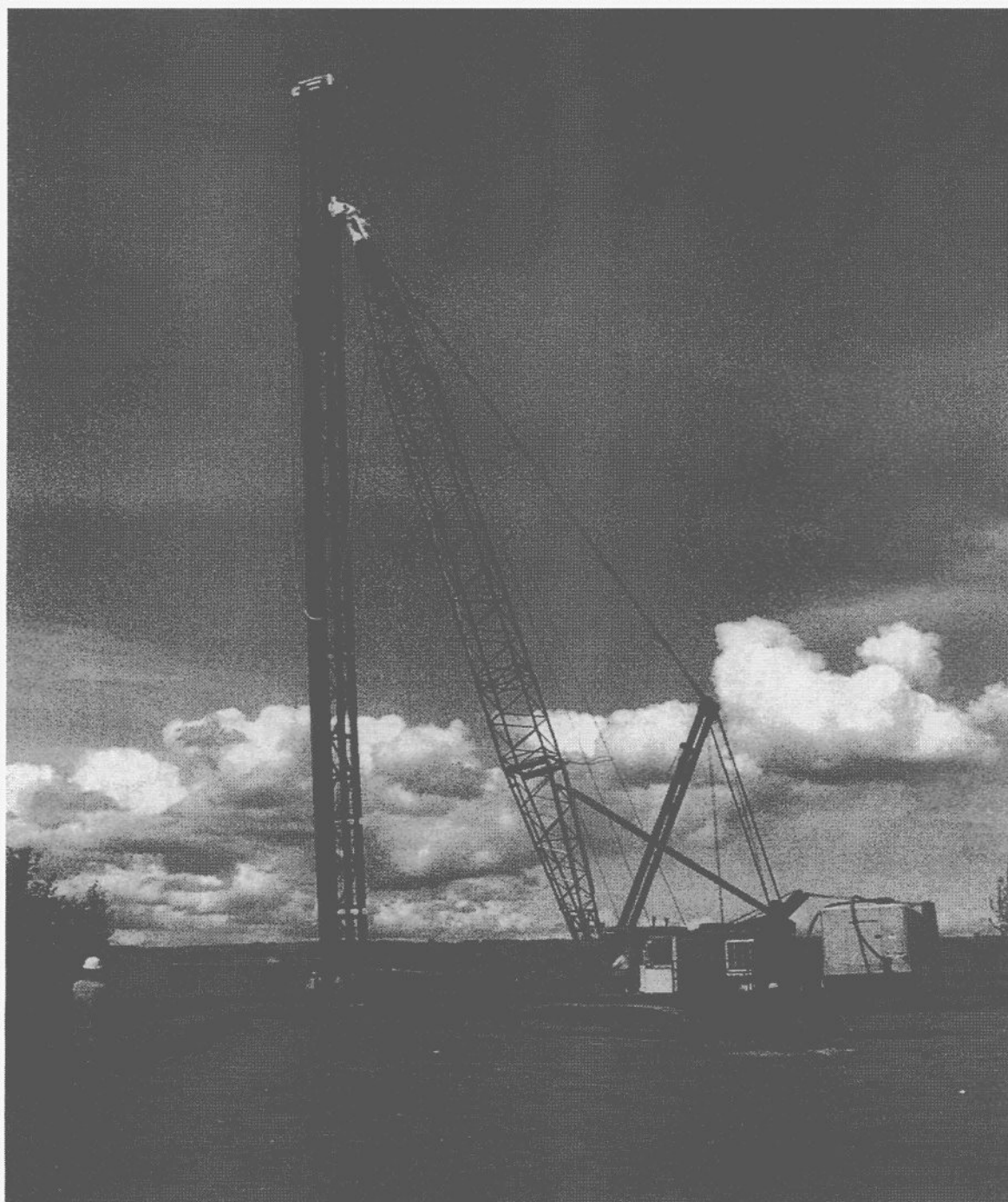
Figure 36-8 The pile driver setup.
