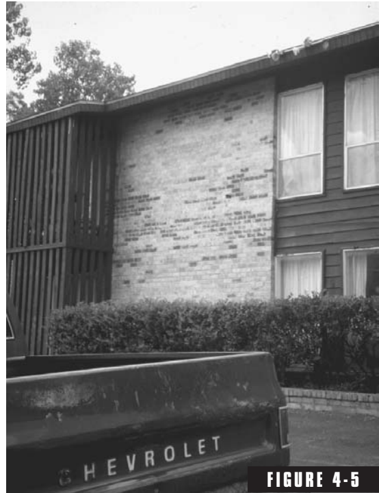
Uneven color distribution. (from Beall, Christine, Masonry Design and Detailing , 4th edition, McGraw-Hill, New York).
