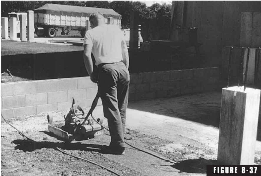
Vibrating plate compactor.
