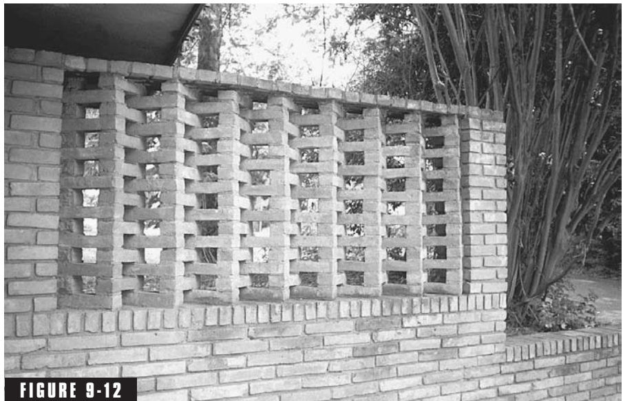
Brick screen walls.
