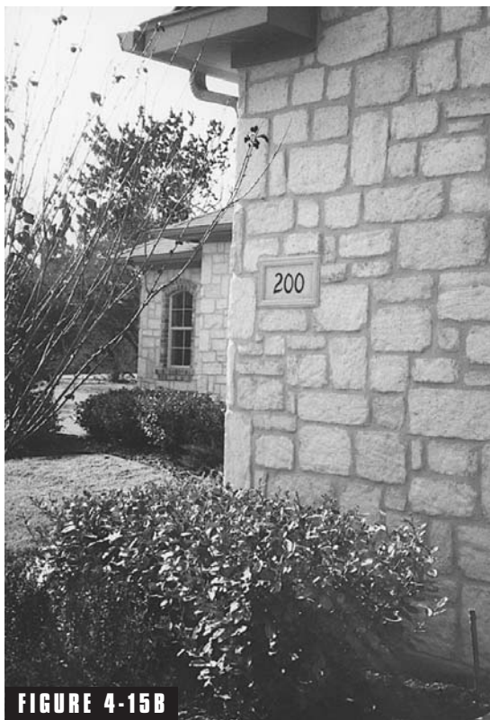
FIGURE 4-15B Cast rubble stone.
