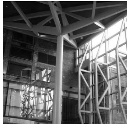
(f) Tree truss column
