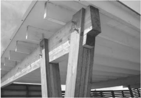
(c) Bolted timber-to-timber connection
