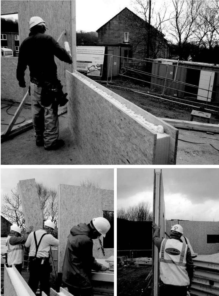
Fig. 1.17. SIPs during construction.
