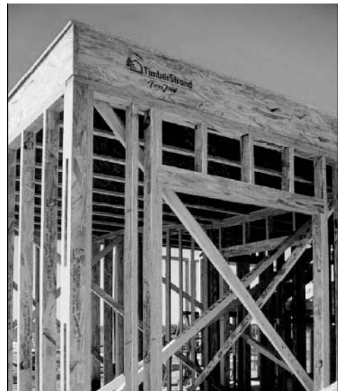
Fig. 1.12. TimberStrand (LSL), courtesy of Weyerhaeuser (iLevel TrusJoist).
