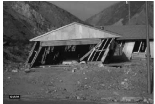
(c) Lack of adequate racking strength results in failure (photo courtesy of APA, The Engineered Wood Association)
