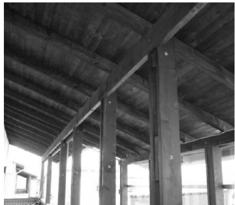
(b) Bolted spaced columns with solid sections
