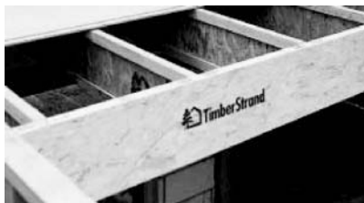
Fig. 1.12. TimberStrand (LSL), courtesy of Weyerhaeuser (iLevel TrusJoist).
