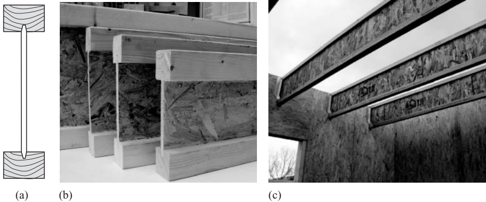
Fig. 1.15. Typical I-joists and their application.
