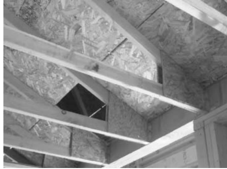
(b) Nailed OSB gusset joints
