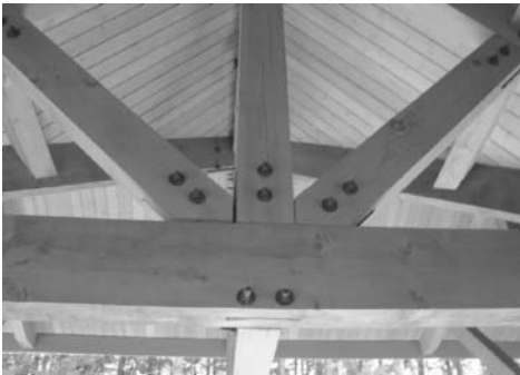
(e) Fin-plate bolted connection (steel plates in slots cut in timber)
