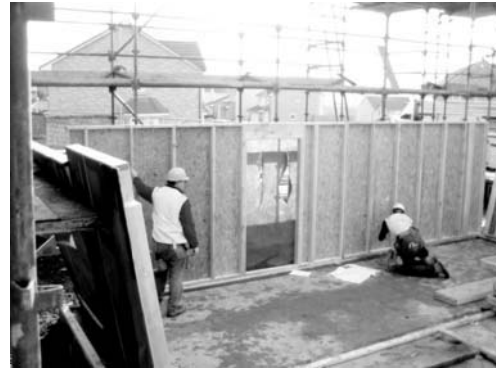
(a) Timber wall during assembly and erection
