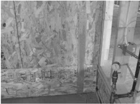
(a) Nailed holding-down strap
