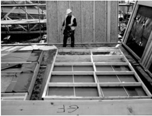
(a) Timber wall during assembly and erection
