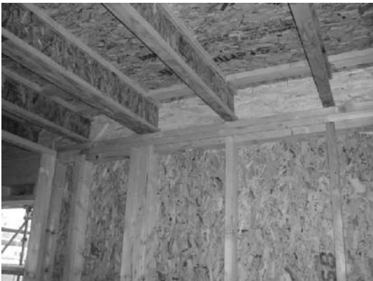
(e) Stud wall – multiple studs to carry higher applied loads
