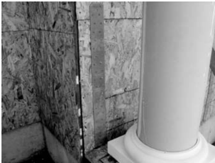
(b) Holding-down strap to prevent overturning
