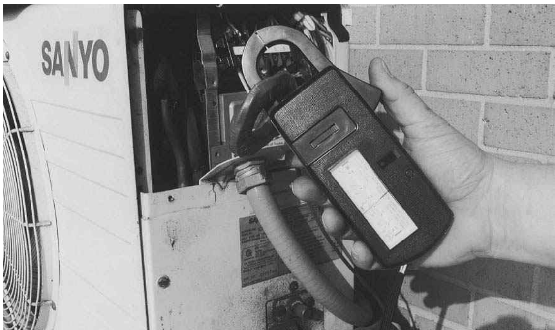
Figure 1-26 A scale divider and clamp-on ammeter being used to measure the control current in an air conditioner.
