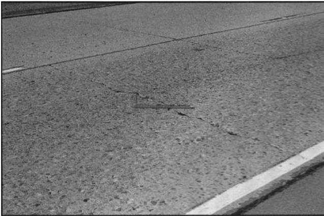
Figure 4.4 High severity transverse crack in JRCP. (From Miller, J.S. and Bellinger, W.Y. 2003. Distress Identification Manual for the Long-Term Pavement Performance Program (Fourth Revised Edition) , FHWA-RD-03-031, p. 41. Washington, DC: Federal Highway Administration, United States Department of Transportation.)
