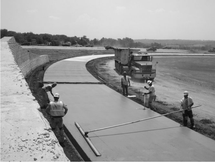
Figure 1.3 Finishing slipformed pavement around a banked curve. (Photo courtesy of The Great Lakes Construction Company, Hinckley, Ohio.)
