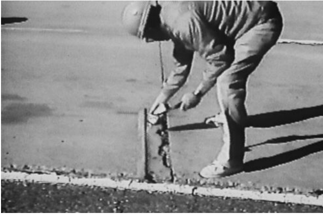
Figure 4.5 High severity transverse joint spalling. (From American Concrete Pavement Association (ACPA) 1996a. Construction of Portland Cement Concrete Pavements, Participant's Manual , FHWA HI-96-027, p. VIII-47. AASHTO/FHWA/INDUSTRY Joint Training, Washington, DC: Federal Highway Administration, United States Department of Transportation. Available on the web at http://isddc.dot.gov/OLPFiles/FHWA/014737.pdf .)
