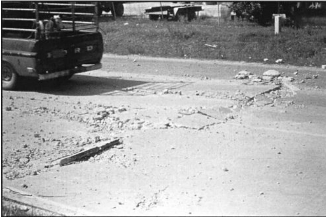
Figure 4.9 Blowup. (From Miller, J.S. and Bellinger, W.Y. 2003. Distress Identification Manual for the Long-Term Pavement Performance Program (Fourth Revised Edition) , FHWA-RD-03-031, p. 52. Washington, DC: Federal Highway Administration, United States Department of Transportation.)
