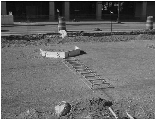
Figure 2.4 Dowel basket assembly with corrosion-resistant epoxy-coated dowels. (Photo by author.)
