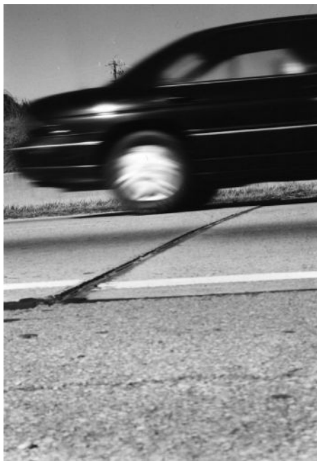
Figure 4.10 Faulted transverse joint. (Photo by author.)
