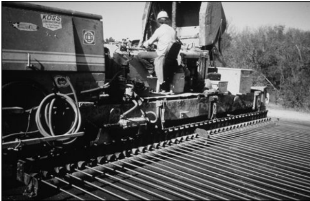
Figure 18.8 CRCP steel installation with tube feeders. (Adapted from American Concrete Pavement Association (ACPA). 1996a. Construction of Portland Cement Concrete Pavements, Participant's Manual , FHWA HI-96-027, AASHTO/FHWA/INDUSTRY Joint Training, Washington, D.C.: Federal Highway Administration, United States Department of Transportation. Available on the web at http://isddc.dot.gov/OLPFiles/FHWA/014737.pdf : VI-37.)
