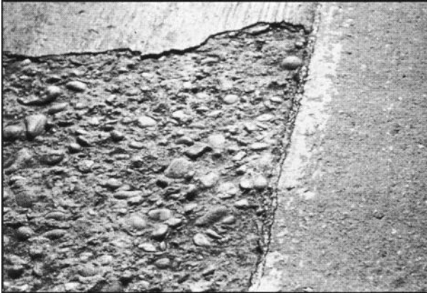
Figure 4.7 Scaling. (From Miller, J.S. and Bellinger, W.Y. 2003. Distress Identification Manual for the Long-Term Pavement Performance Program (Fourth Revised Edition) , FHWA-RD-03-031, p. 48. Washington, DC: Federal Highway Administration, United States Department of Transportation.)
