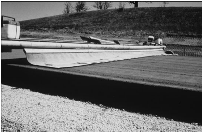
Figure 19.2 Burlap drag to provide microtexture. (Adapted from American Concrete Pavement Association (ACPA). 1996a. Construction of Portland Cement Concrete Pavements, Participant's Manual , FHWA HI-96-027, AASHTO/FHWA/INDUSTRY Joint Training, Washington, D.C.: Federal Highway Administration, United States Department of Transportation. Available on the web at http://isddc.dot.gov/OLPFiles/FHWA/014737.pdf : VI-53.)
