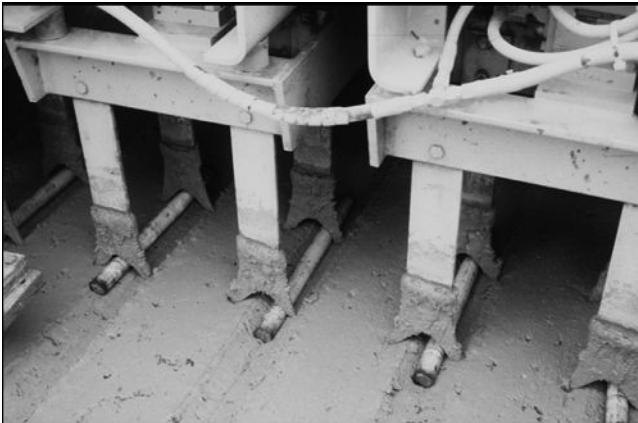
Figure 18.7 Dowel bar inserters. (Adapted from American Concrete Pavement Association (ACPA). 1996a. Construction of Portland Cement Concrete Pavements, Participant's Manual , FHWA HI-96-027, AASHTO/FHWA/INDUSTRY Joint Training, Washington, D.C.: Federal Highway Administration, United States Department of Transportation. Available on the web at http://isddc.dot.gov/OLPFiles/FHWA/014737.pdf : VI-32.)
