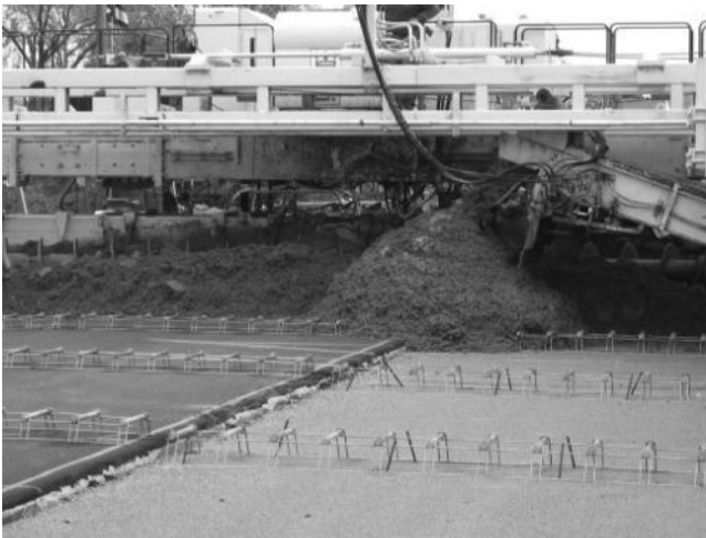
Figure 22.3 Unbonded overlay on two lanes with a third lane paved at the same time. (Photo courtesy: Dale Crowl.)
