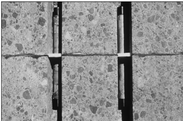
Figure 21.4 Dowel bar retrofit. (From American Concrete Pavement Association (ACPA). 1996a. Construction of Portland Cement Concrete Pavements, Participant's Manual , FHWA HI-96-027, AASHTO/FHWA/INDUSTRY Joint Training, Washington, D.C.: Federal Highway Administration, United States Department of Transportation. Available on the web at http://isddc.dot.gov/OLPFiles/FHWA/014737.pdf : VIII-66.)
