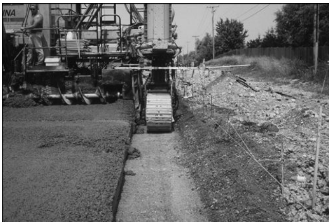
Figure 18.4 The pad line. (Adapted from American Concrete Pavement Association (ACPA). 1996a. Construction of Portland Cement Concrete Pavements, Participant's Manual , FHWA HI-96-027, AASHTO/FHWA/INDUSTRY Joint Training, Washington, D.C.: Federal Highway Administration, United States Department of Transportation. Available on the web at http://isddc.dot.gov/OLPFiles/FHWA/014737.pdf : VI-20.)
