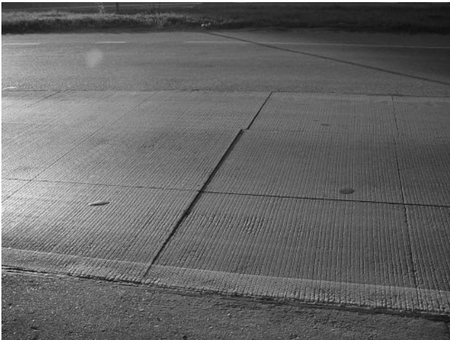
Figure 22.9 Failure of UTW by panel sliding. (Photo by the author).
