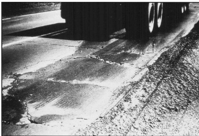
Figure 4.11 Water bleeding and pumping. (From Miller, J.S. and Bellinger, W.Y. 2003. Distress Identification Manual for the Long-Term Pavement Performance Program (Fourth Revised Edition) , FHWA-RD-03-031, p. 58. Washington, DC: Federal Highway Administration, United States Department of Transportation.)
