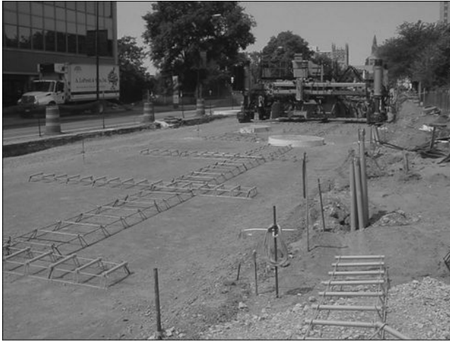
Figure 2.6 Tie bar basket assemblies with corrosion-resistant epoxy-coated tie bars—dowel baskets are also shown. (Photo by author.)
