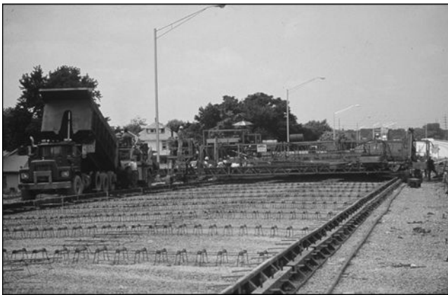
Figure 18.9 Fixed-form paving. (Adapted from American Concrete Pavement Association (ACPA). 1996a. Construction of Portland Cement Concrete Pavements, Participant's Manual , FHWA HI-96-027, AASHTO/FHWA/INDUSTRY Joint Training, Washington, D.C.: Federal Highway Administration, United States Department of Transportation. Available on the web at http://isddc.dot.gov/OLPFiles/FHWA/014737.pdf : VI-68.)
