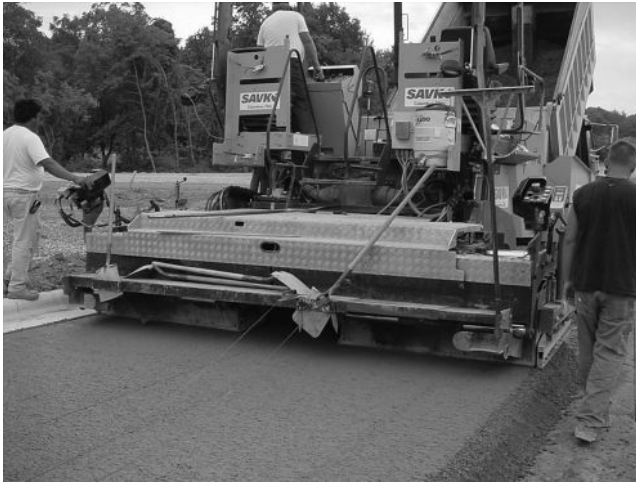
Figure 2.10 RCC pavement construction—Columbus, Ohio. (Photo by author.)
