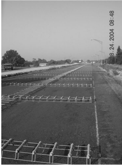
Figure 1.1 Dowel and tie bar baskets placed in preparation for slipform paving. (Photo courtesy of The Great Lakes Construction Company, Hinckley, Ohio.)
