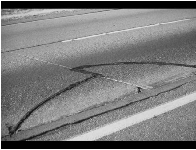
Figure 4.1 Corner breaks. (From American Concrete Pavement Association (ACPA) 1996a. Construction of Portland Cement Concrete Pavements, Participant's Manual, FHWA HI-96-027 , p. VIII-16. AASHTO/FHWA/INDUSTRY Joint Training, Washington, DC: Federal Highway Administration, United States Department of Transportation. Available on the web at http://isddc.dot.gov/OLPFiles/FHWA/014737.pdf .)
