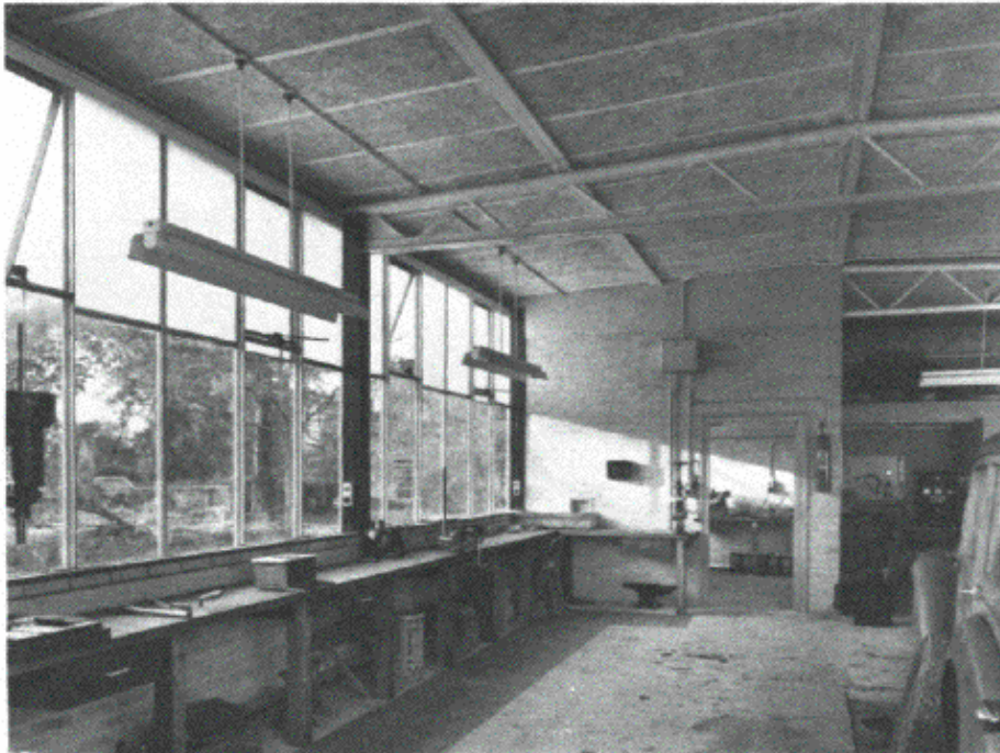
Figure 1 Have the materials stood the test of time? The architects had no reply when asked this question by their clients when this farm workshop was being built in 1955. They had specified some of the promising materials of the post-war period: short bored piles, flint lime bricks, light steel trusses, woodwool decking, three layers roof felt and aluminium patent glazing with some laminated insulating glass. Fortunately it has survived 35 years with only the roof felt requiring replacement in 1989 and it is still in use as a workshop. Nowadays the durability question should be settled at the briefing stage. Architects: Stillman and Eastwick-Field.
