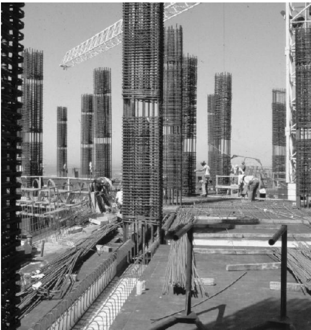
PHOTO 4.2 Installation of reinforcing bars in the Pacific Park Plaza building (courtesy of Mr. James Tai, T.Y. International, San Francisco).
