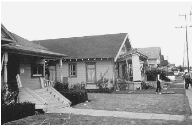
FIGURE 7.5 Houses damaged due to cripple wall failure, 1983 Coalinga Earthquake (courtesy of EQE International).
