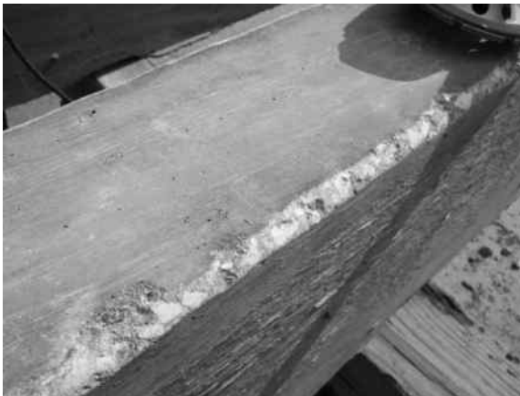
FIGURE 8.5 Rounded beam corners by grinding.
