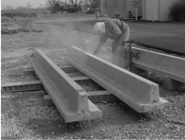
FIGURE 8.4 Surface preparations by sandblasting.
