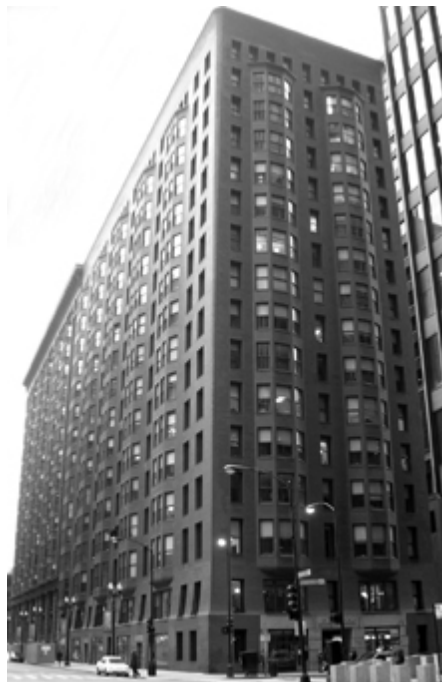
FIGURE 1.1 Monadnock Building, Chicago, USA, 1891
