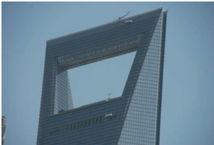
FIGURE 6.11 Shanghai World Financial Center, aerodynamic top (courtesy of Niels Jakob Darger)
