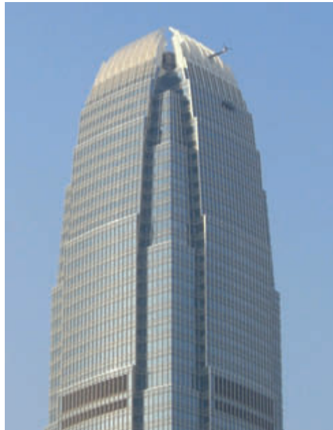
FIGURE 6.9 Two International Finance Centre, aerodynamic top (courtesy of Antony Wood/CTBUH)
