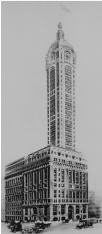
FIGURE 1.4 Singer Building, New York, USA, 1908
