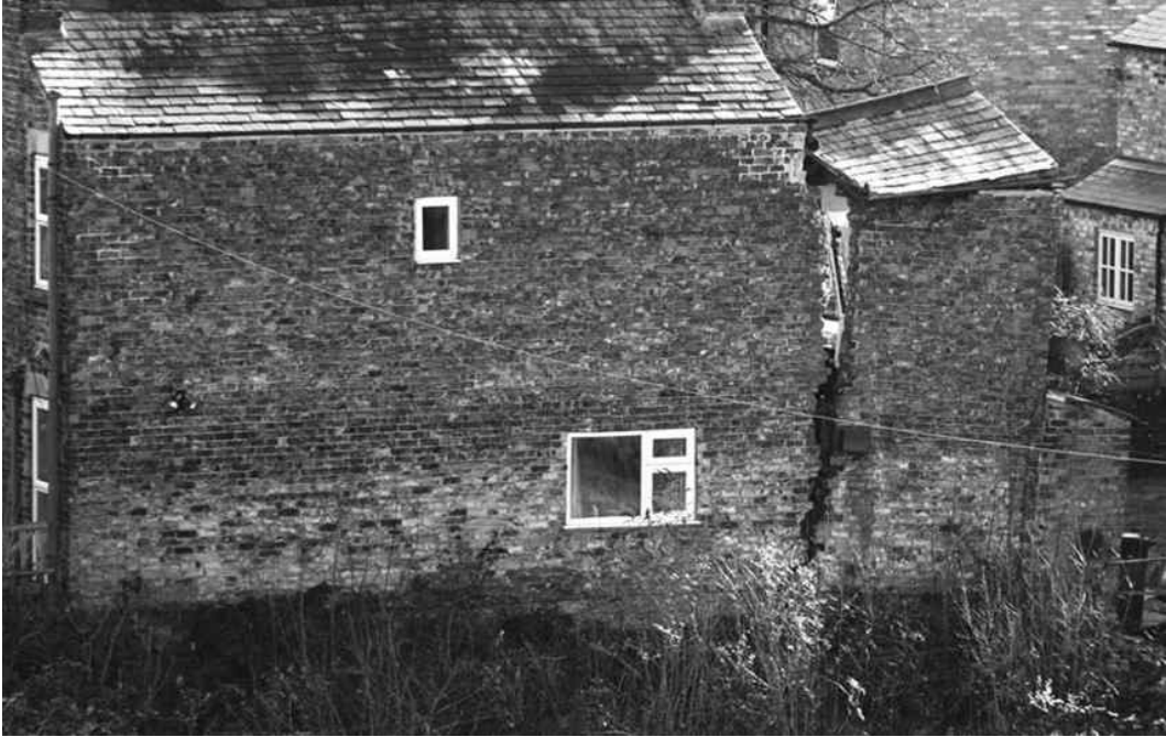
Figure 12.1: Photograph showing damage caused by a sinkhole in Ripon, Yorkshire. By kind permission of The Press, York.
