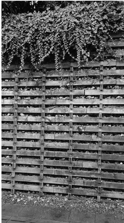
Figure 16.6: Photograph showing a typical crib wall construction.
