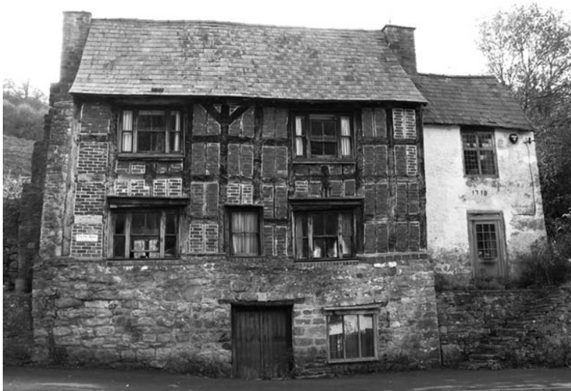
Figure 3.8: A timber frame building circa 1500s with an extension to the right-hand side dated 1718.
