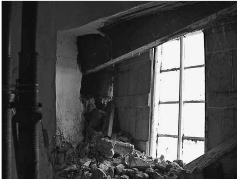
Figure 18.4: Photograph showing the loss of bearing of a beam subject to wet-rot deterioration.
