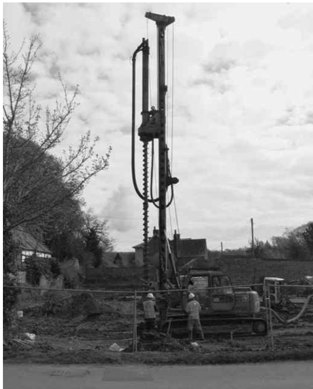
Figure 7.6: Photograph showing a bored pile foundation activity.
