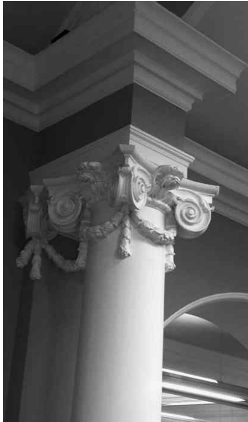
Figure 11.10: Photograph showing a Corinthian column.
