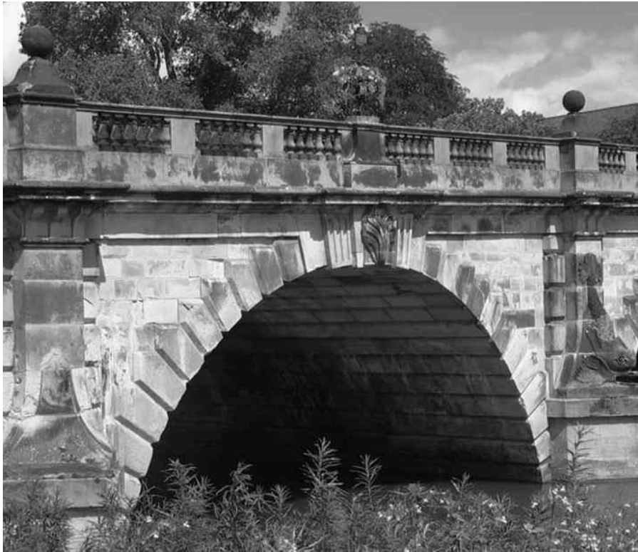
Figure 11.1: Photograph showing the keystones and voussoirs running through the length of the English Bridge at Shrewsbury in the formation of the arch.
