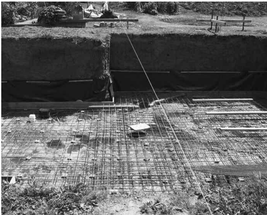
Figure 16.8: Showing the commencement of a basement structure.
