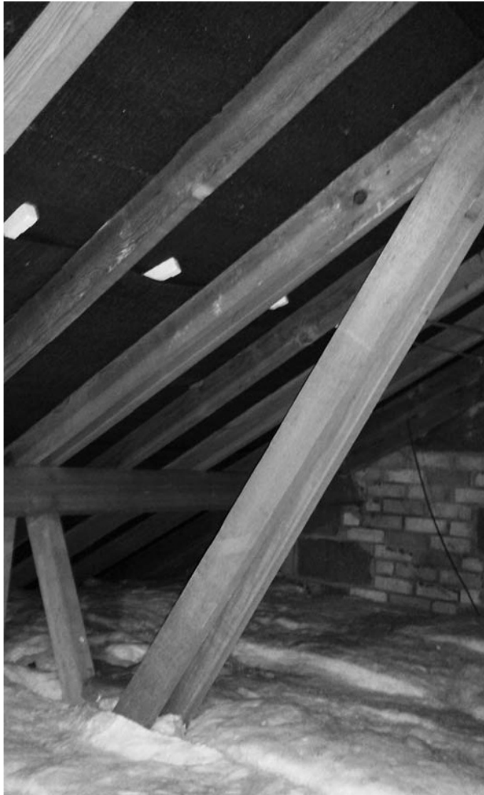
Figure 1.11: Photograph of a TRADA truss.
