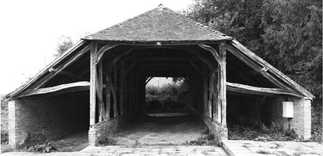
Figure 3.20: An aisled barn construction.
