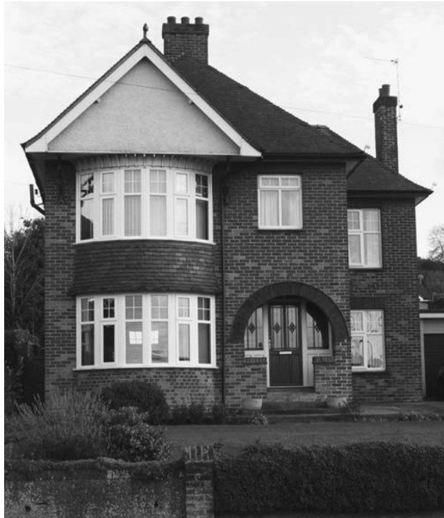
Figure 1.9: Photograph showing a typical 1930s property.
