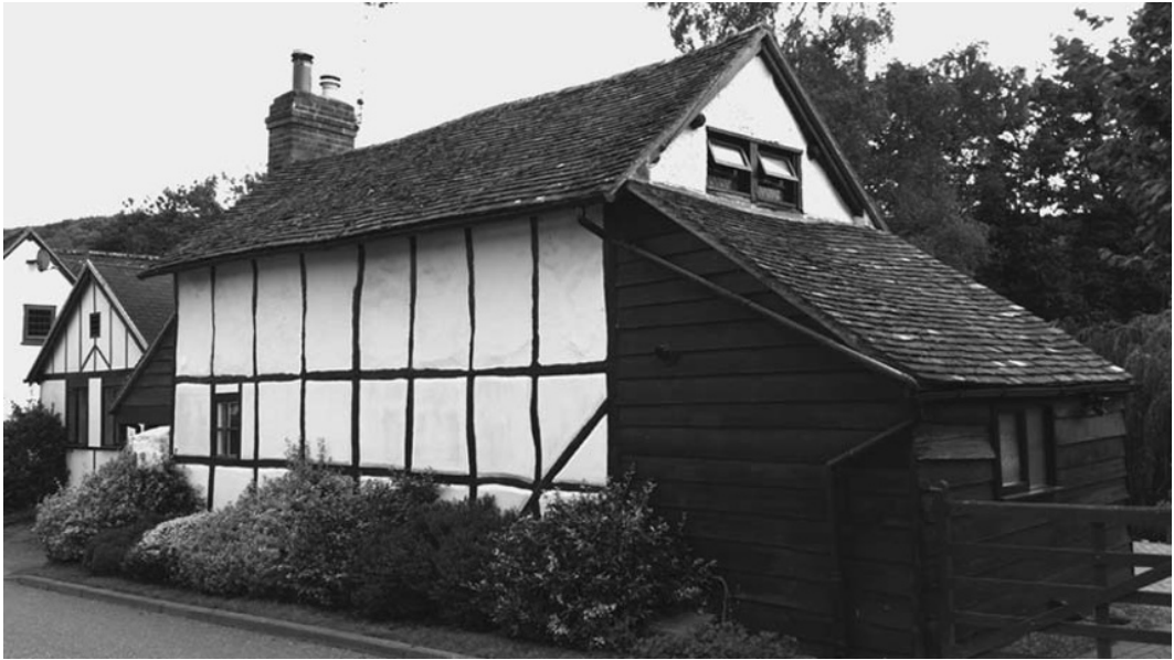
Figure 3.11: A traditional timber frame from the 1700s.
