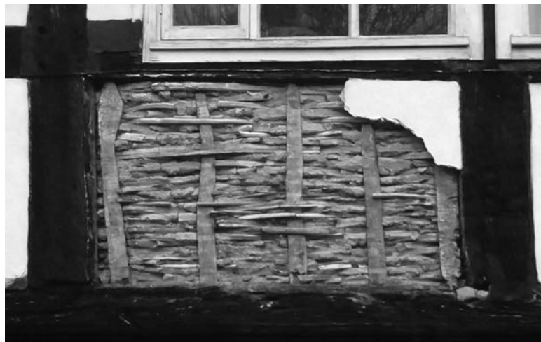
Figure 3.13: Photograph showing wattle and daub exposed on a damaged property in Herefordshire.
