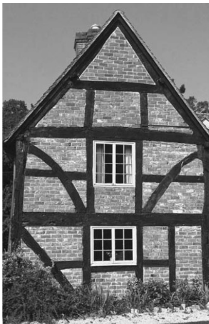
Figure 3.10: A property constructed circa 1600s with convex knee brace and queen post truss.
