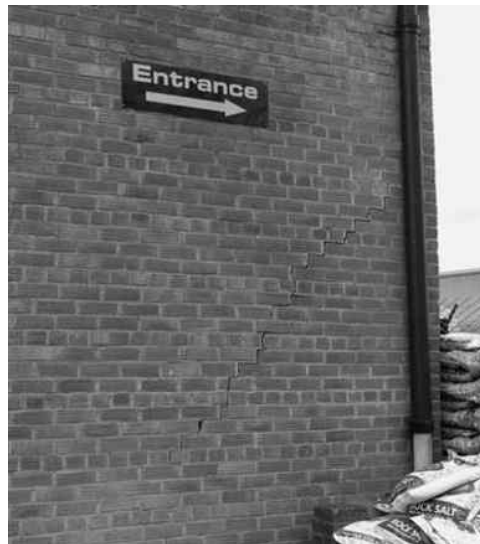
Figure 18.2: Photograph showing diagonal subsidence crack in a building.
