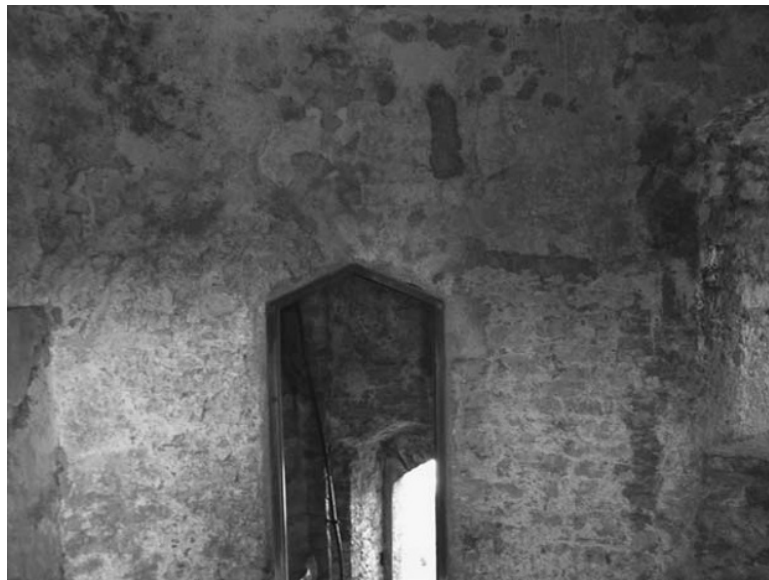
Figure 3.22: Photograph of lime-washed walls at Pembroke Castle.
