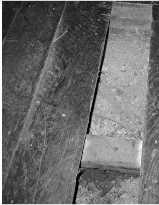
Figure 9.1: Photograph showing a timber floor laid directly onto earth in a Georgian property.
