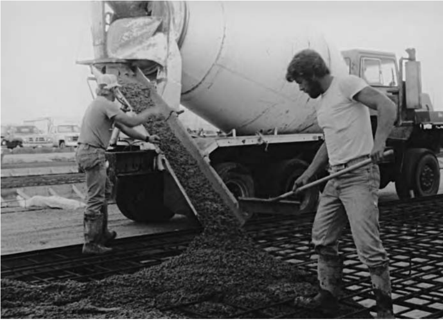
Figure 7.1 A slump of about 100–125 mm (4–5 in), as shown here, often works well in slab construction
