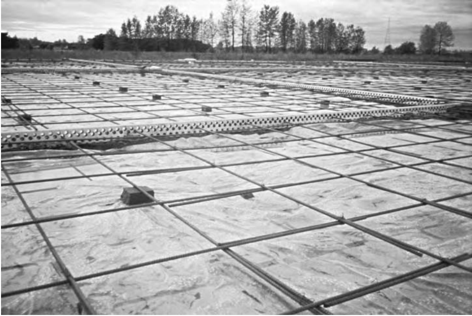
Figure 16.3 Light reinforcement for crack control in a jointed slab – 12-mm (#4) bars spaced 600 mm (24 in) on centre
