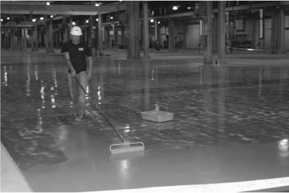
Figure 21.1 An epoxy coating resists many forms of chemical attack
