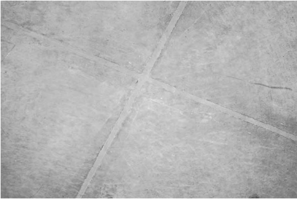
Figure 15.6 Warehouse floor joints filled with semi-rigid epoxy
