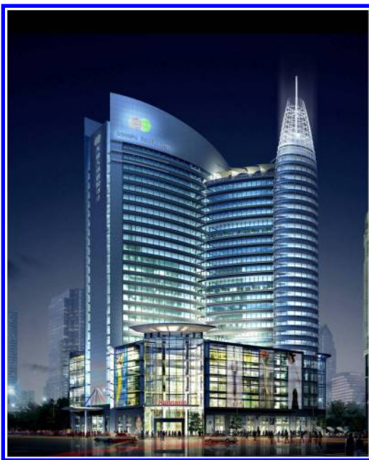
Picture 7. Tianyin Mansion in Guangzhou.
