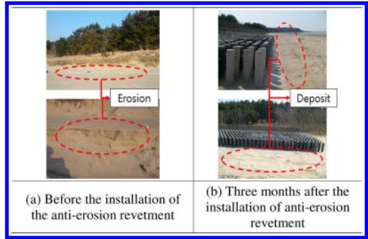
Figure 14. Before and after the installation of the anti-erosion revetment.
