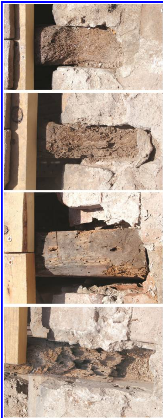
Figure 5. Rafters: V-19, V-20, V-21 and V-22.
