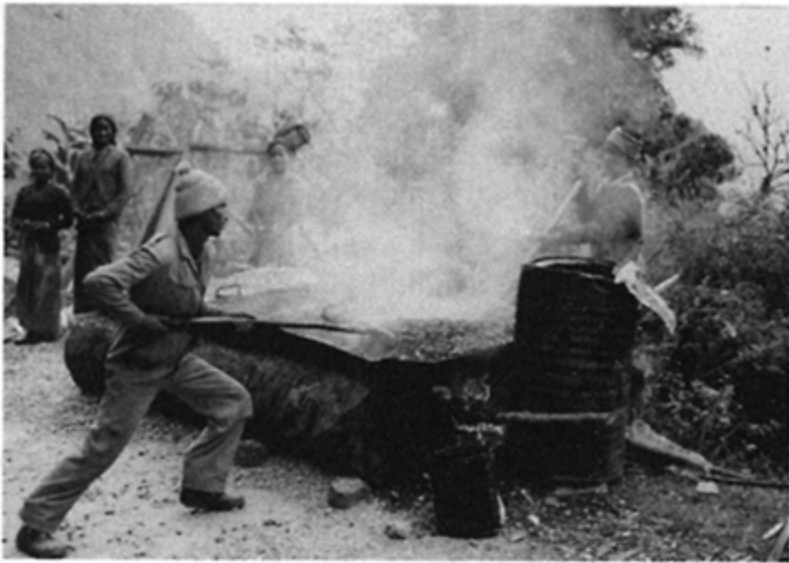
Figure 19.4 Hand-mixing hot asphalt in India.
