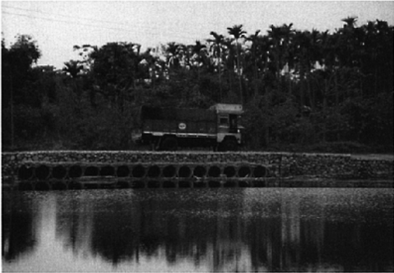
Multiple culvert in India (Photo by Bent Thagesen)
