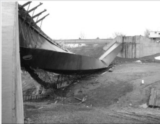
Fig. CS1 Cross-section of Marcy Bridge and the failure due to lateral-torsional buckling (source: Corr, et al, 2009)
