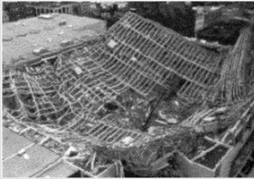
(c) View of the collapsed roof
