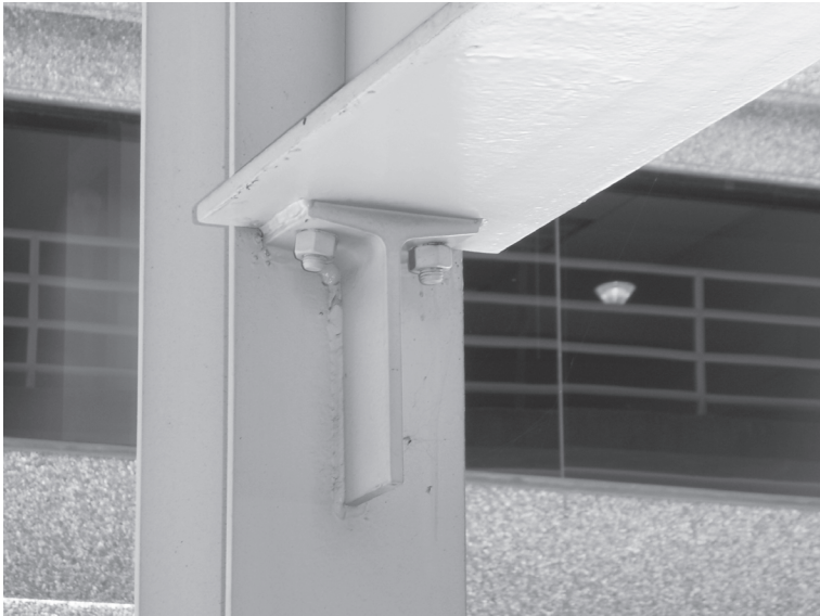
Fig. 11.33 Welded stiffened seat connection using the split I-section in a car parking structure in Bethesda, USA. (The bolts are erection bolts.)
