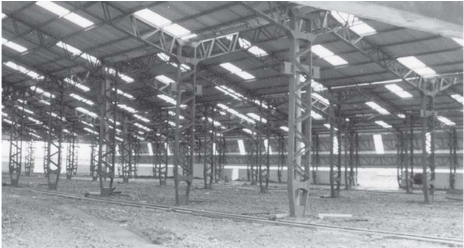
Built-up column in a portal frame, Mumbai (Note the stubs in the column, which carry a small crane).
