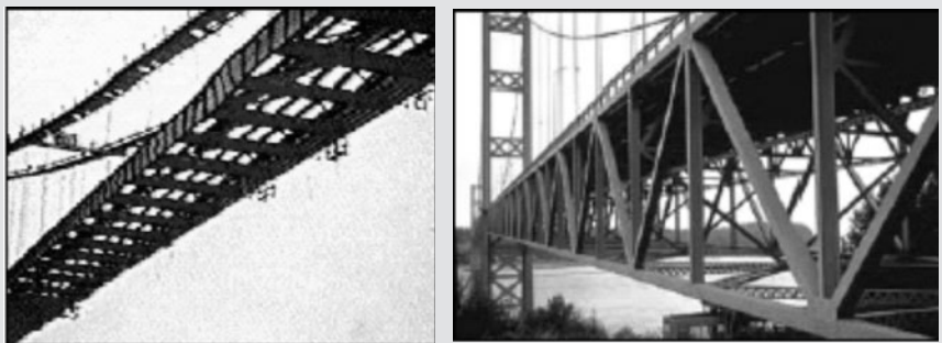
Fig. CS2 Solid I-beams in the deck of the original bridge and trussed deck of the reconstructed bridge ( www.failurebydesign.info )
