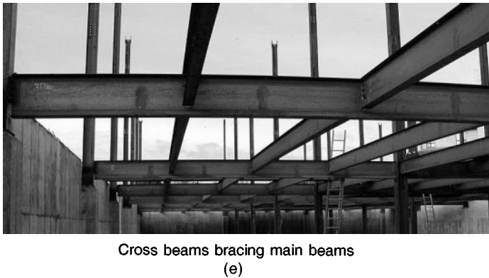
Fig. 6.4 Lateral bracing systems for roof and floor beams
