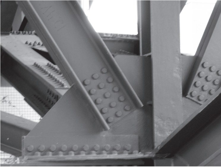
Fig. 10.16 Example of a connection using HSFG bolts
