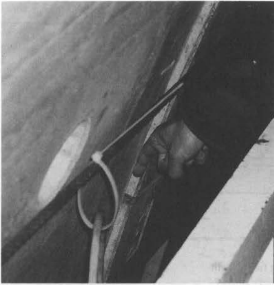
Figure 7.33 Differential displacement as observed at the Second Heinenoord tunnel
