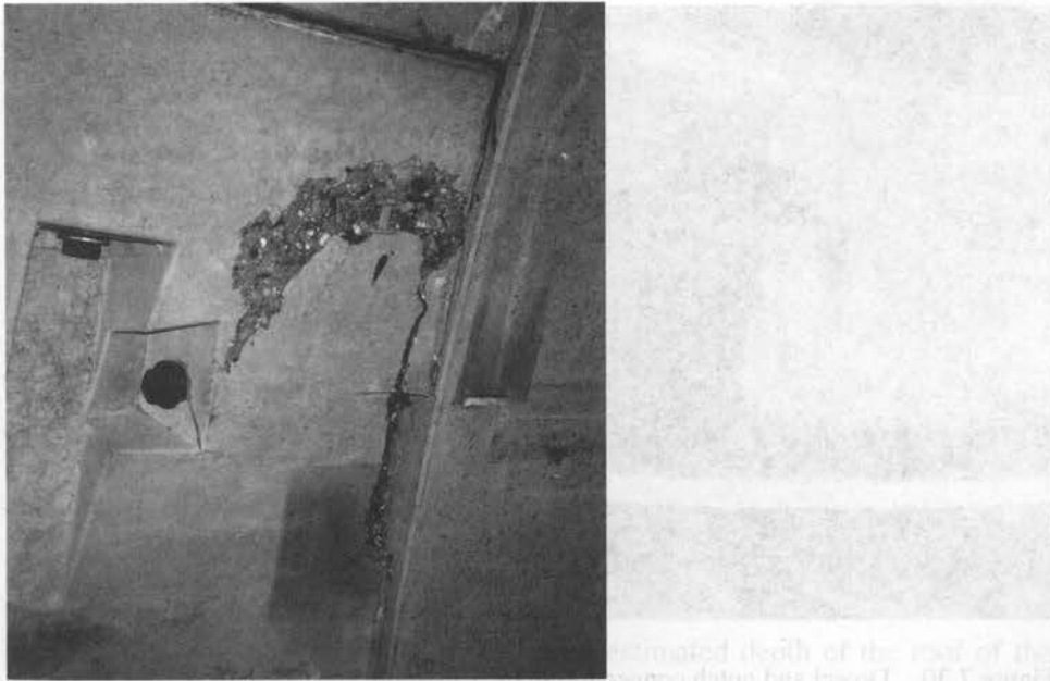
Figure 7.29 Damage to the tunnel lining; i.e. damage near the dowel and notch system
