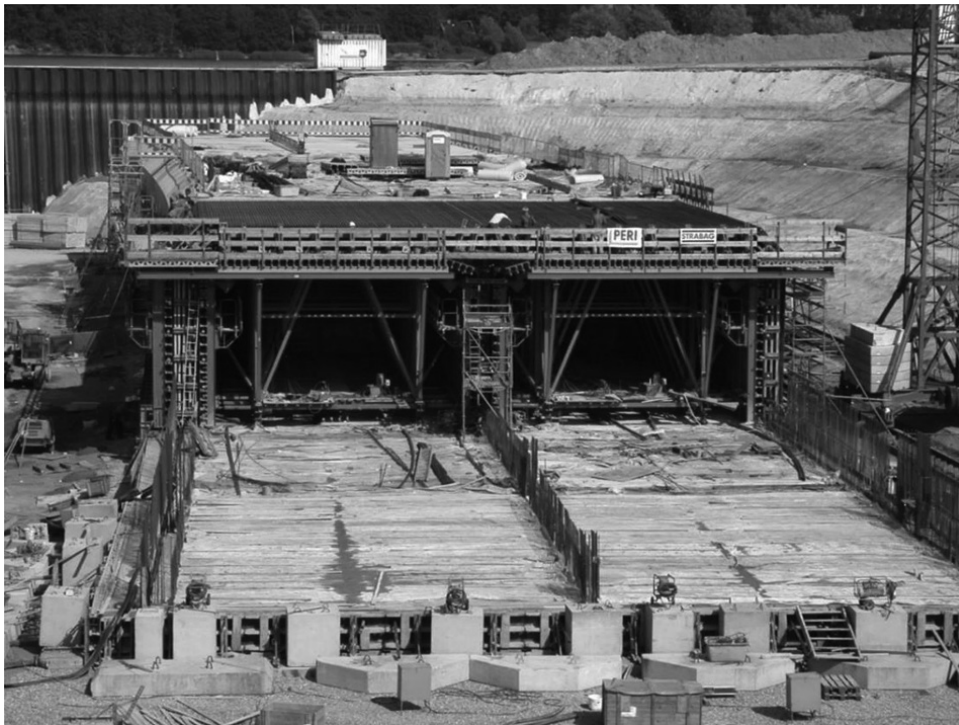
Figure 2.26 Assembly of tunnel segments
