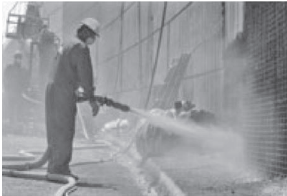
FIGURE 8.16 Using shotcrete.
