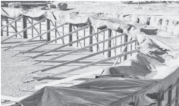
FIGURE 6.18 Plastic sheet to protect from evaporation.
