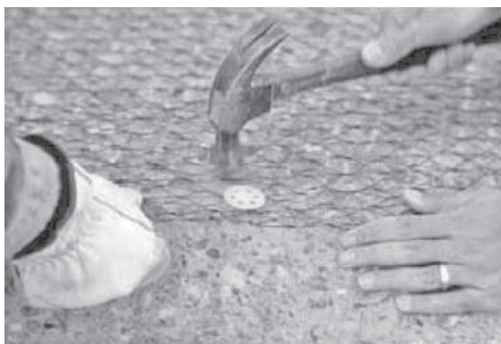
FIGURE 7.15b Fixing titanium mesh by plastic binder.
