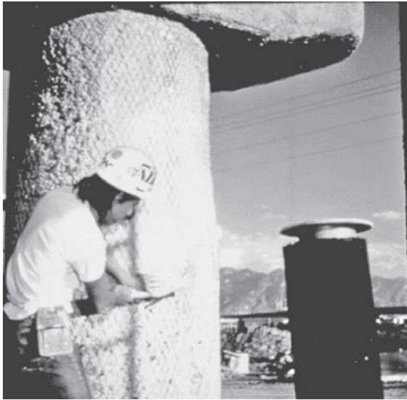
FIGURE 7.11 Fixing titanium on a concrete column.
