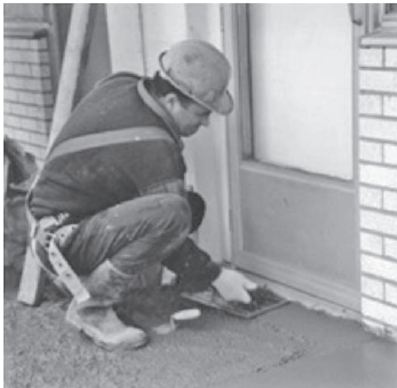
FIGURE 8.13 Manual method for repair.
