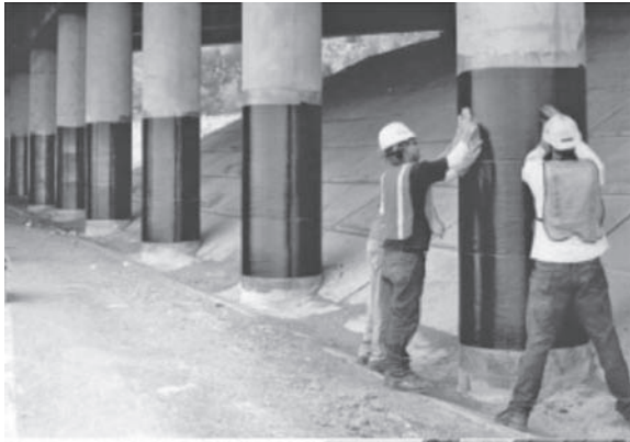
FIGURE 8.27 Column repair.
