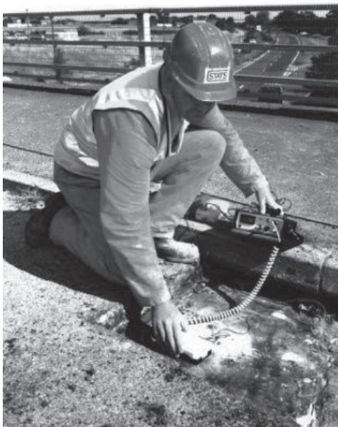
FIGURE 4.22 Concrete cover measurement to a bridge deck.
