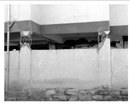
Fig. 11.7 Poorly compacted concrete due to congestion of reinforcement at the top of columns
