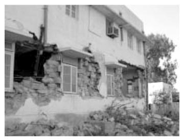
Fig. 11.4 Failure of a typical stone masonry building
