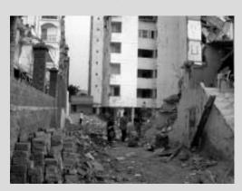
Fig. 11.6 Failure due to soft storey
