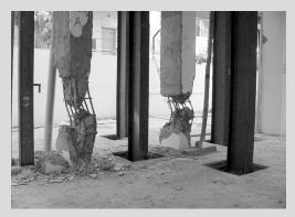
Fig. 11.5 Column failures due to non-ductile detailing
