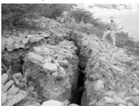
Fig. 11.3 Failure on upstream face of earthen dam
