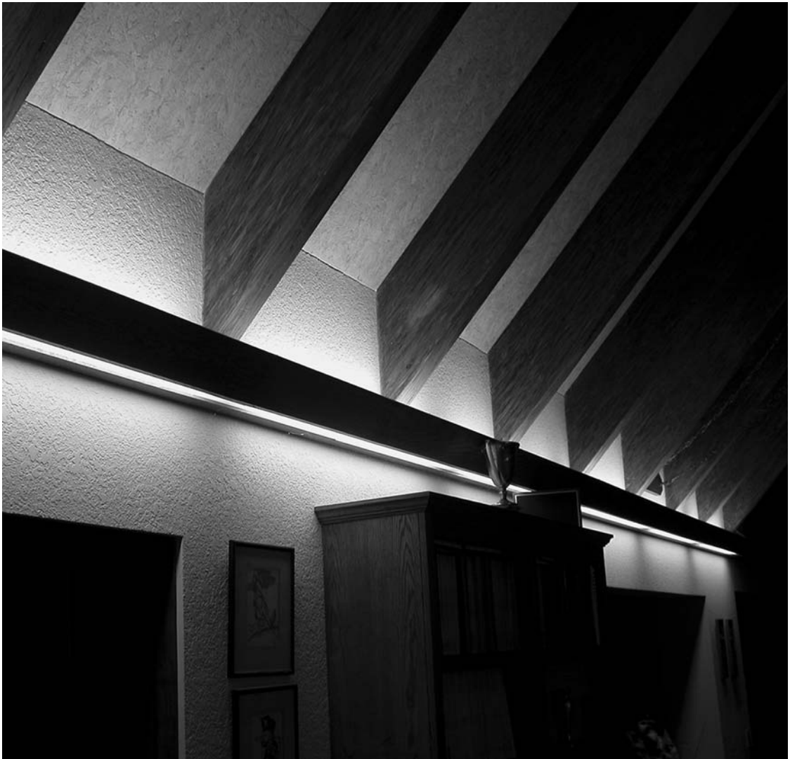
Figure 7.13 Photograph showing soffit lighting of ceiling rafters.
