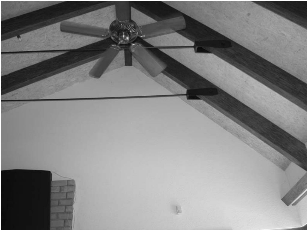
Figure 7.3 Exposed beam ceiling inside of 45° slope roof.
