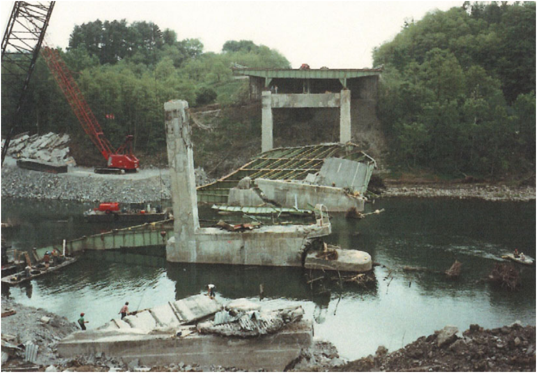
Figure 1-4. Schoharie Creek Bridge collapsed spans.
