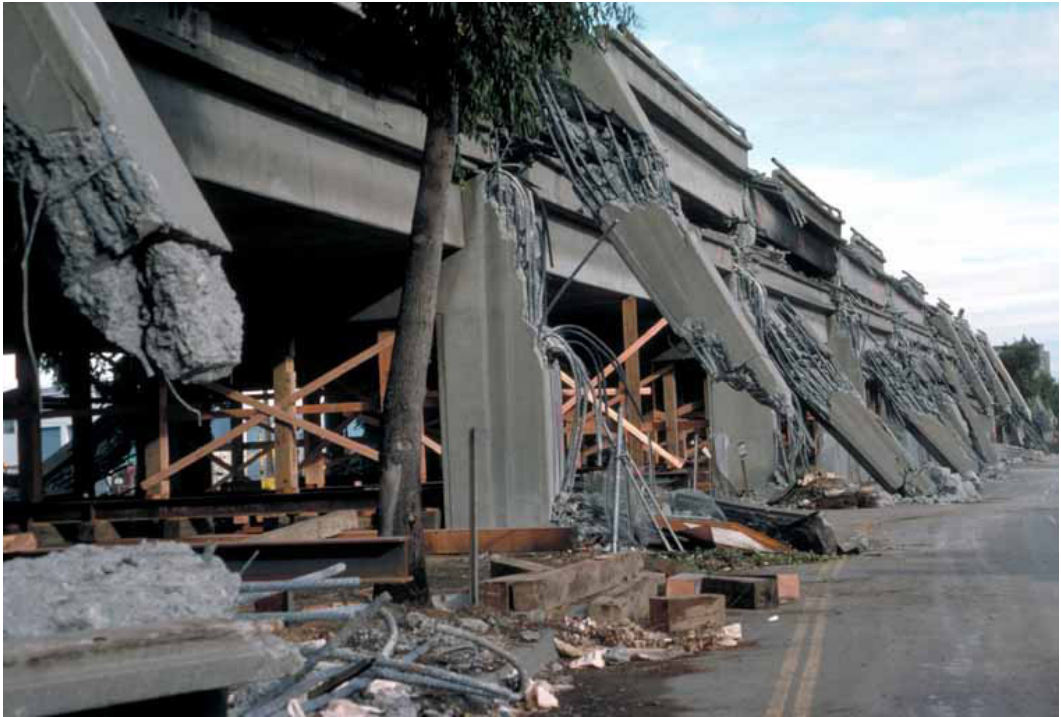
Figure 4-4. Cypress Viaduct Support Column Failure.
