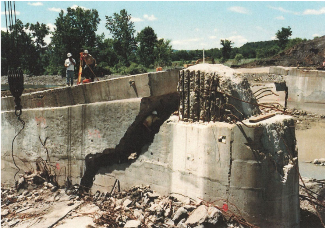
Figure 1-5. Schoharie Creek Bridge failed plinth.
