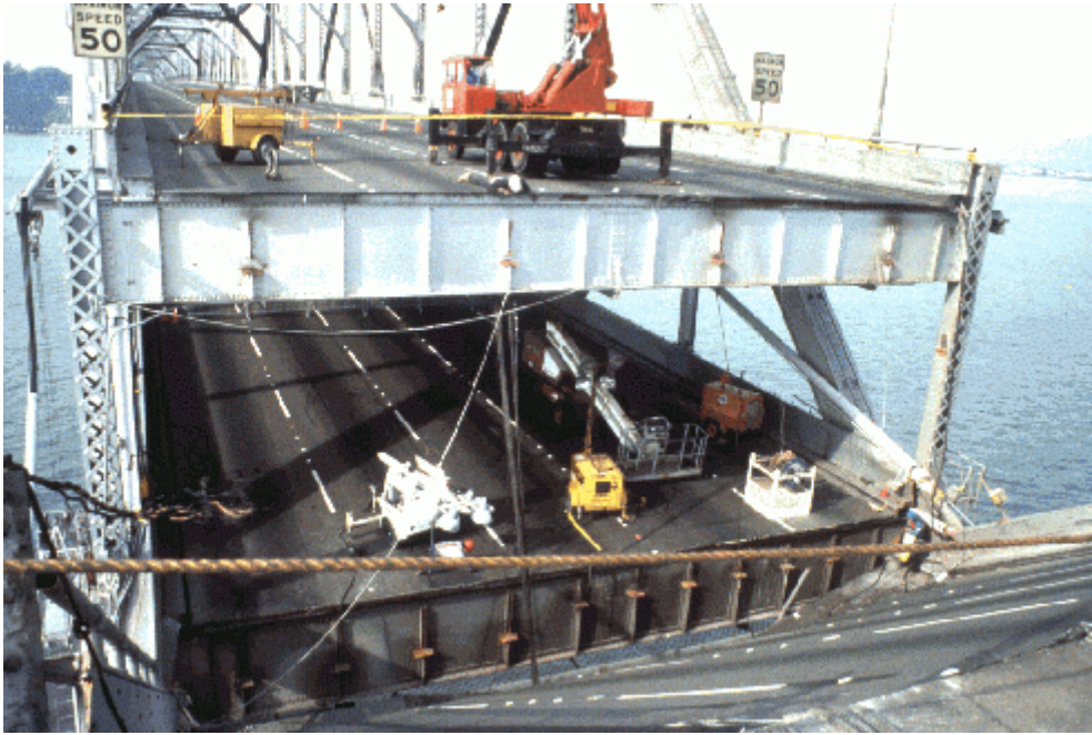
Figure 4-3. Damage to San Francisco-Oakland Bay Bridge.
