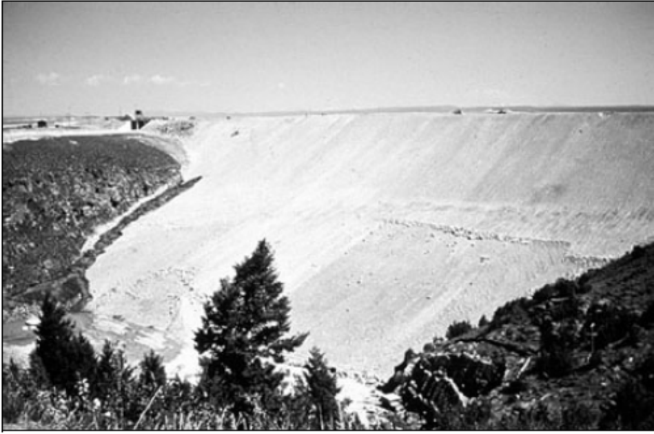
Figure 2-6. Teton Dam Failure Sequence, Initial Erosion.
