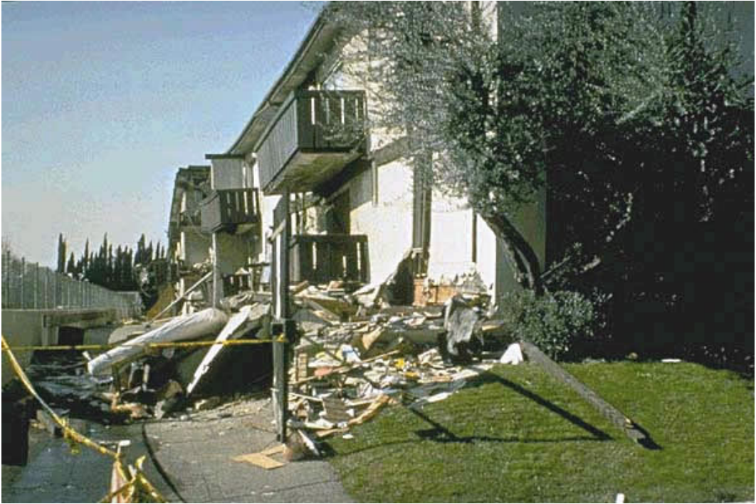
Figure 5-20. Collapsed first floor of Northridge Meadows Apartment.
