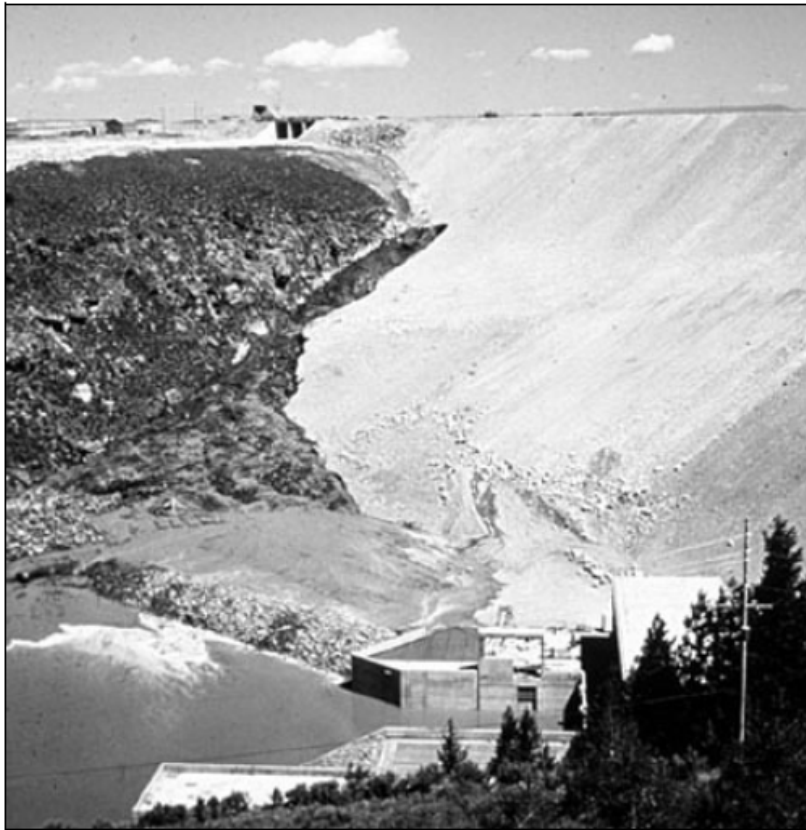
Figure 2-7. Teton Dam Failure Sequence, the Seepage Widens.
