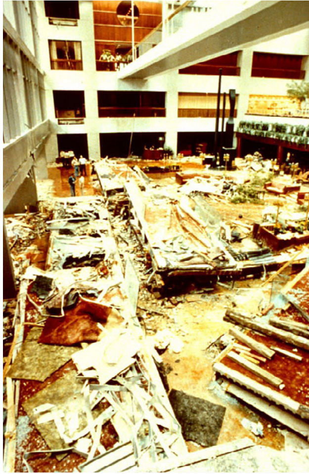
Figure 5-13. Second and Fourth Floor Skywalks collapsed in lobby. Source: Courtesy of Wiss, Janney, Elstner Associates, Inc.
