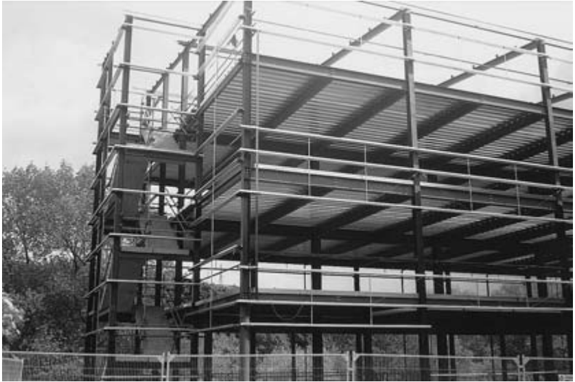
Fig. 22.1 Steel-framed office building under construction.
