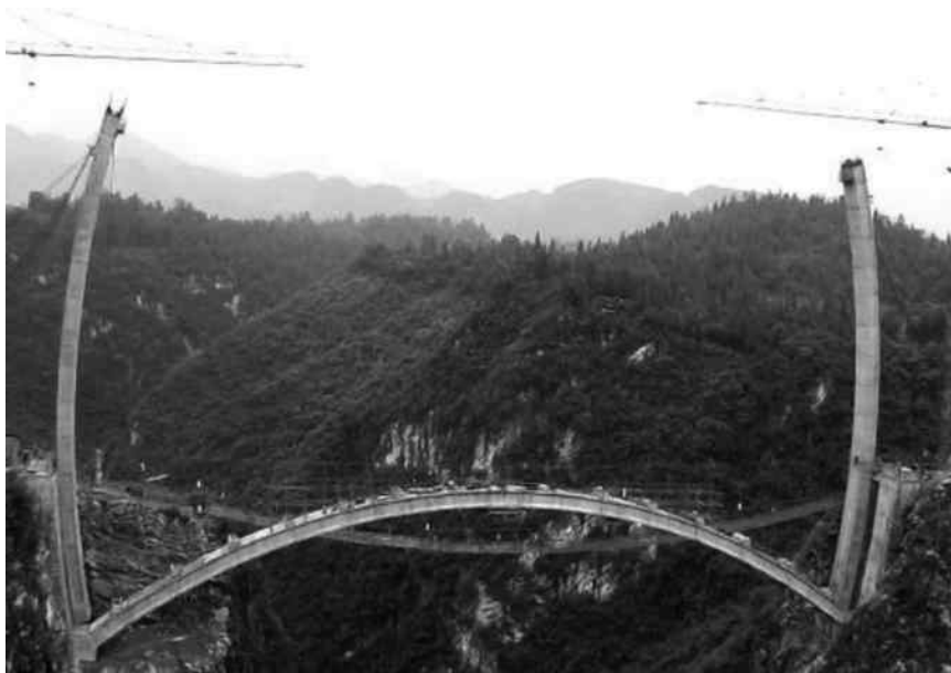
Figure 9.6 Vertical casting and rotating of arch bridge. (Zhenzhu Bridge, China, 2008, Courtesy of Guizhou Bridge Construction Group Ltd.)
