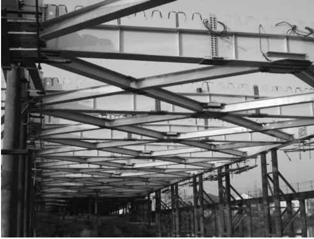
Figure 10.36 Rigid connections of Shang Xin Bridge.
