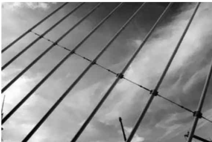
Figure 11.7 Crosstie of cables.
