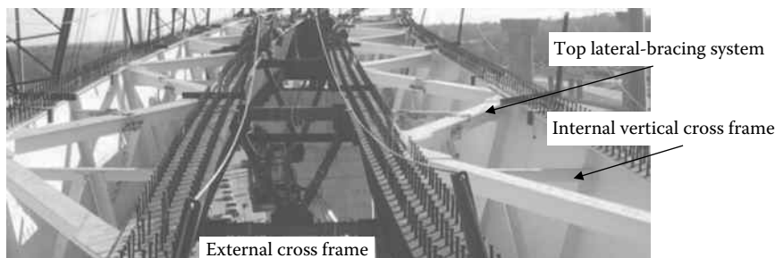
Figure 8.2 Twin-box girder bridge. (Courtesy of TXDOT.)
