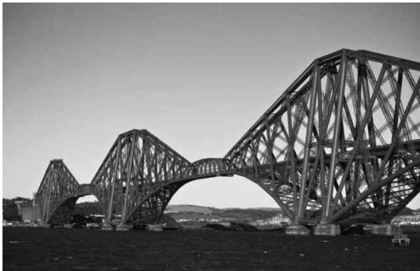
Figure 10.7 Forth Rail Bridge, Queensferry, Scotland.
