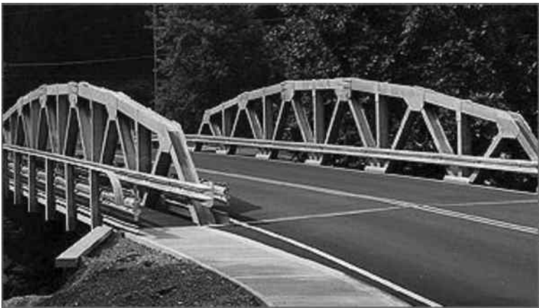
Figure 14.8 Pony truss bridge.
