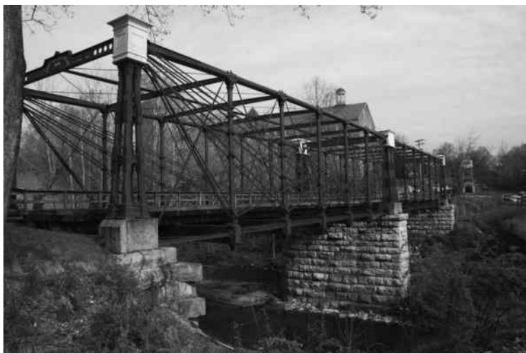
Figure 10.2 Bollman truss bridge.
