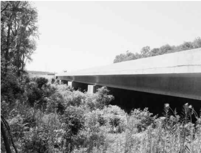
Figure 5.32 US23043 Bridge, Maryland.
