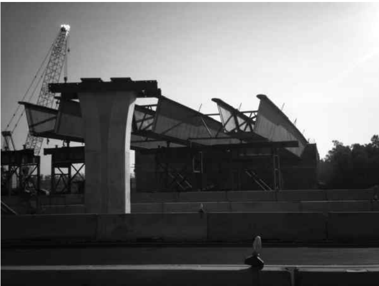
Figure 8.22 Estero Parkway Bridge constructed as a three-span continuous bridge.
